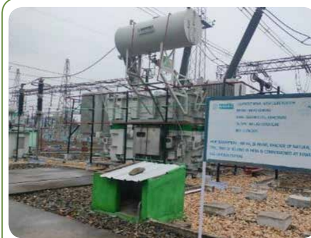
MAITHON SUBSTATION WITH REACTOR CONTAINING ESTER OIL
