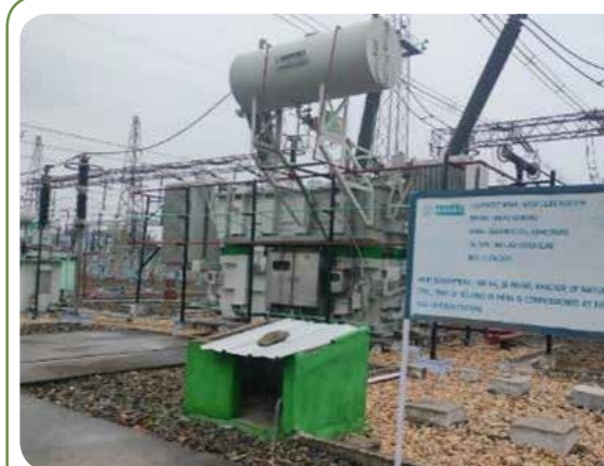
MAITHON SUBSTATION WITH REACTOR CONTAINING ESTER OIL
