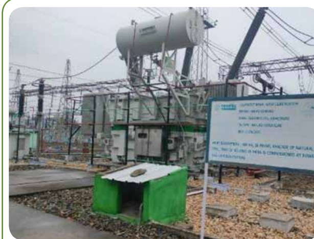
MAITHON SUBSTATION WITH REACTOR CONTAINING ESTER OIL
