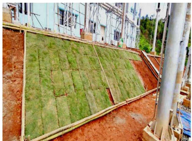
**Grass with bamboo grids (Bio-engineering measures) for slope protection/ soil stabilization work under progress at 220/132 Mawngap & 220/132/33 kV GIS Substation New Shillong**
