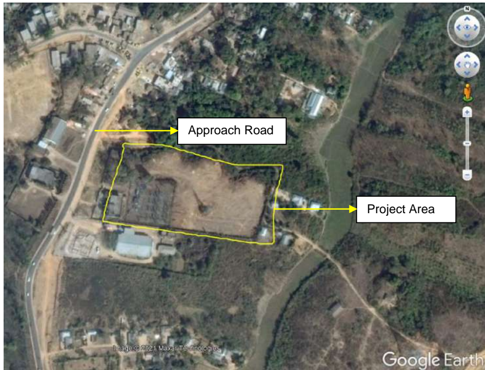
S/S Site in 2017 Before Construction
