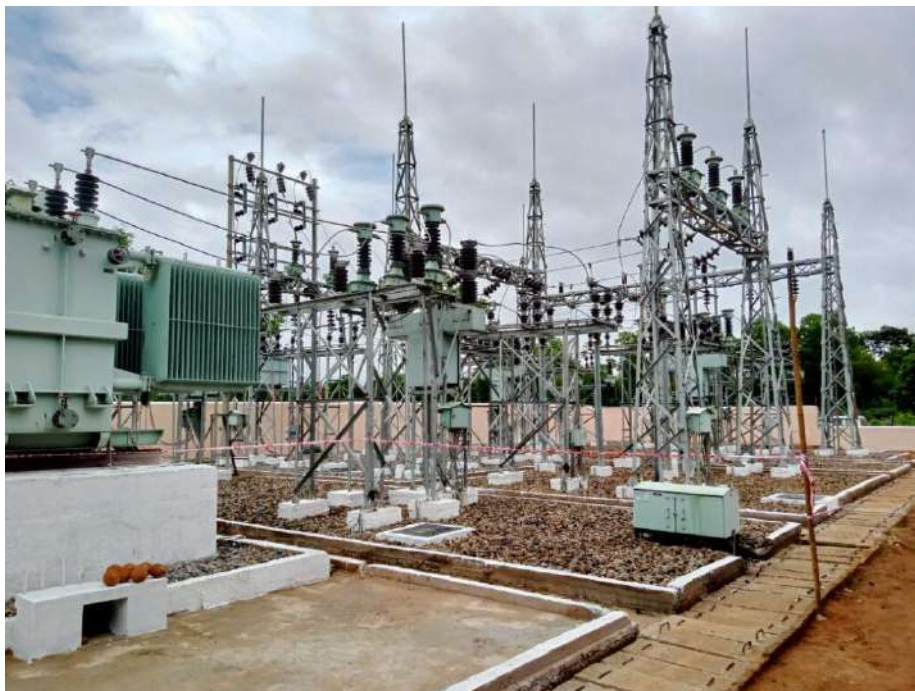
Transformer and Transmission Tower Erection at Simna S/S – Construction Completed
