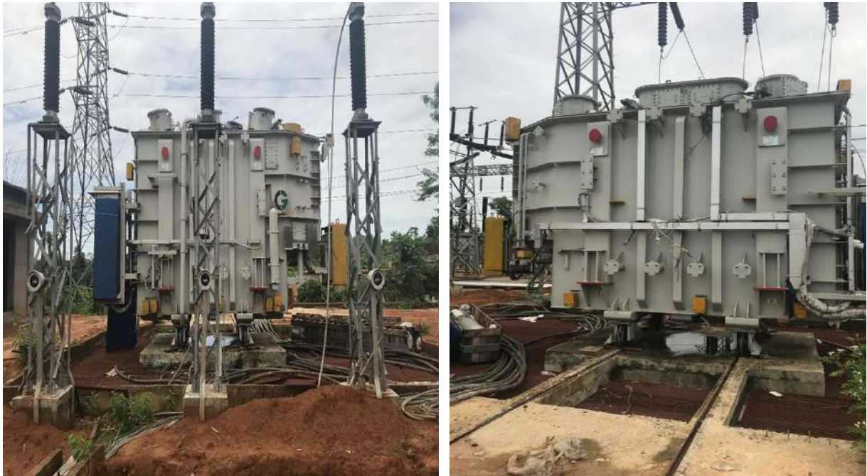
Transformer Erection and Oil Collection Pit at Gokul Nagar S/S Site
