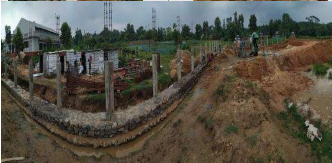
Retention Wall at 132 / 33kV Belonia SS
