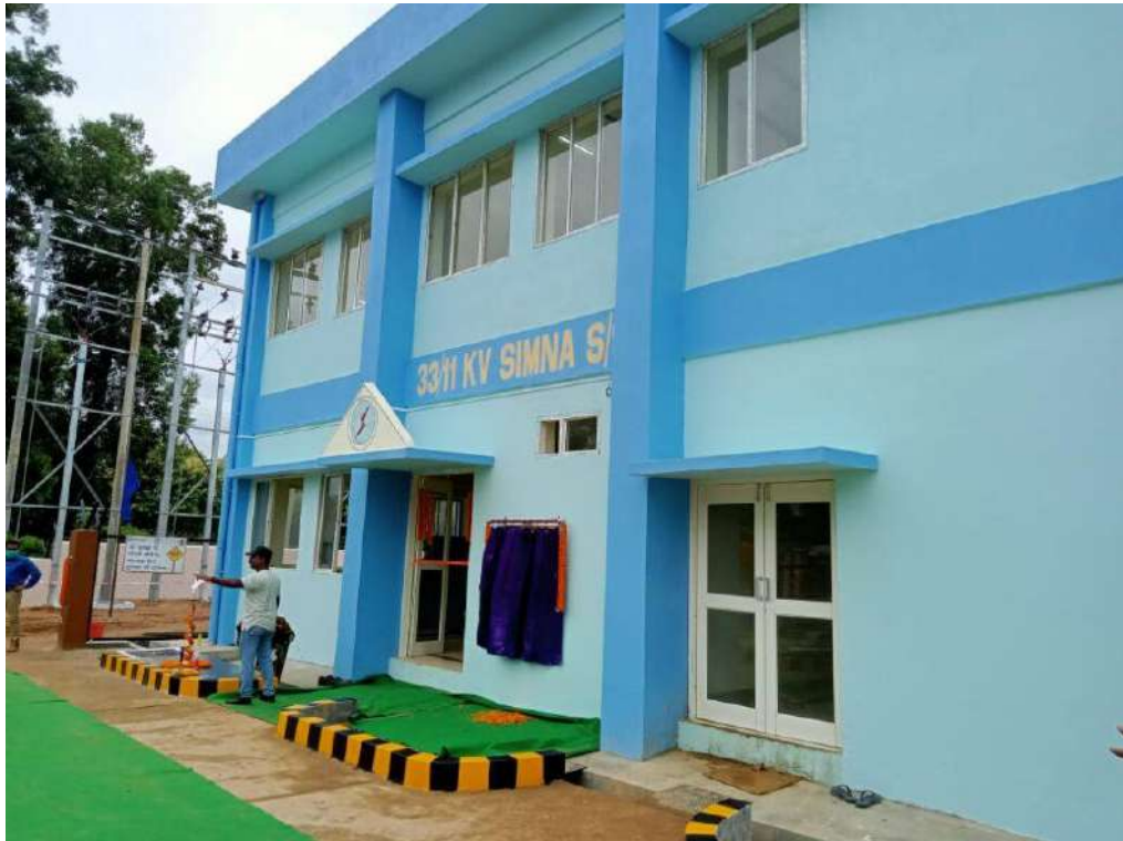
Control Room Building – Simna S/S – Construction Completed
