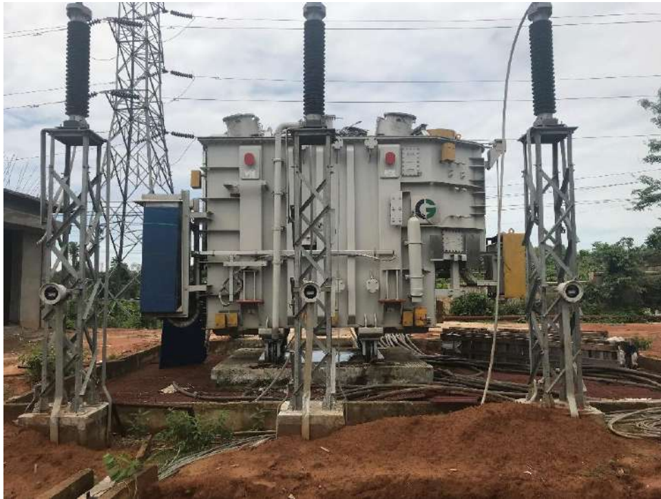
Transformer Erection with Oil Pit – Gokul Nagar S/S
