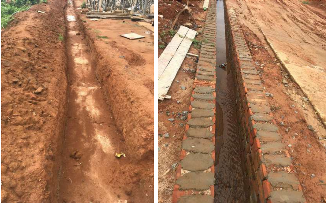
Drainage Channel Construction in Progress at Gokul Nagar S/S
