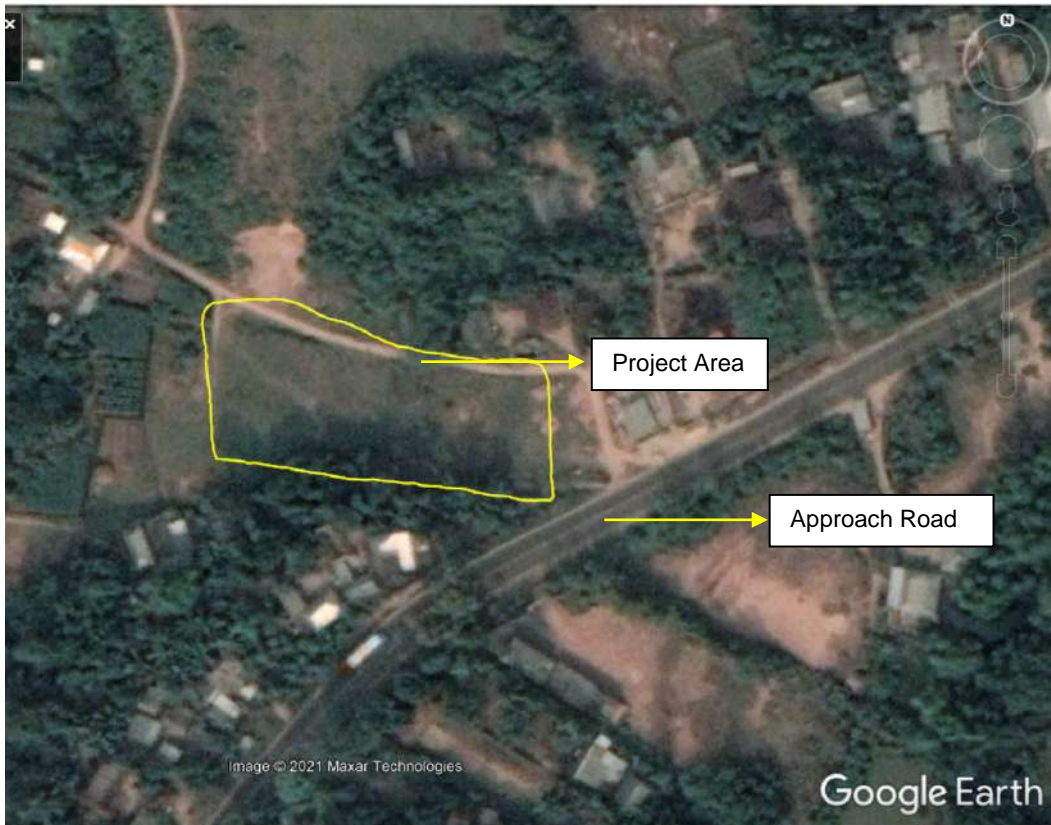
S/S Site in 2021 – Construction Work in Progress. Image is not available for 2021
