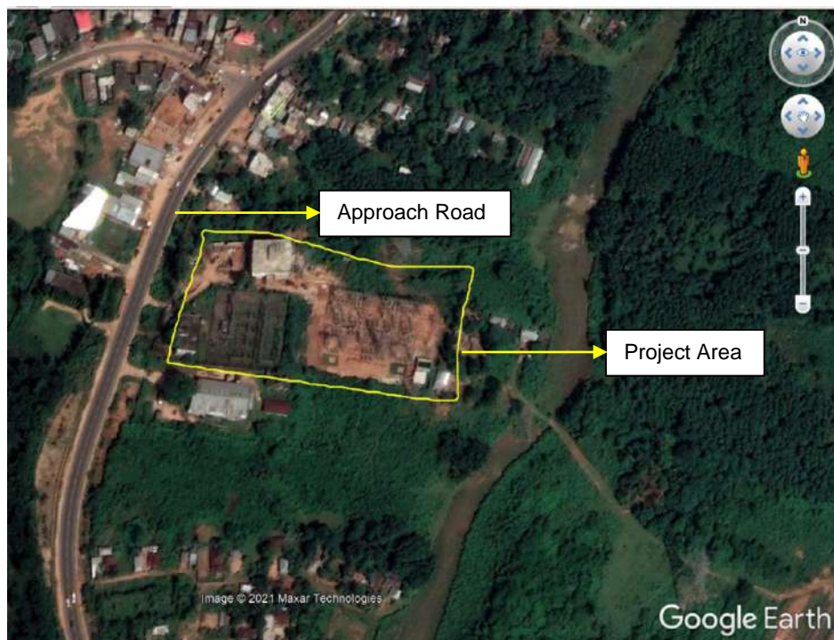
S/S Site in 2021 – Construction Completed
