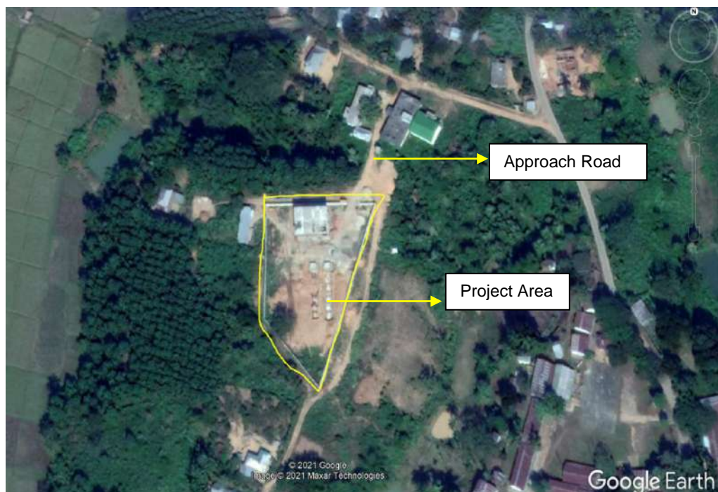
S/S Site in 2021 – Construction Completed (Line test charged on 10.01.2020)
