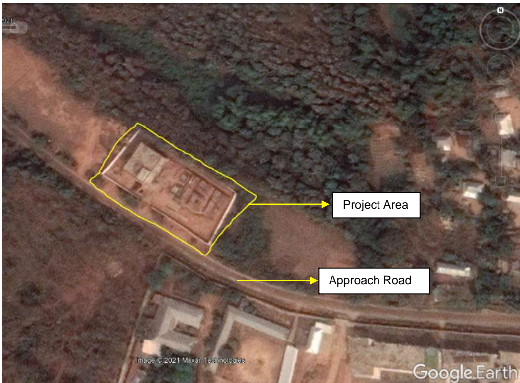
S/S Site in 2021 – Construction Completed
