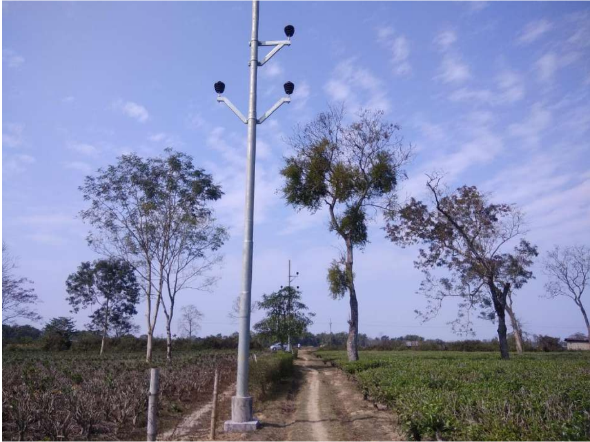
Figure 5-7: Example of Pole erection where Tree is Prevented from Cutting
