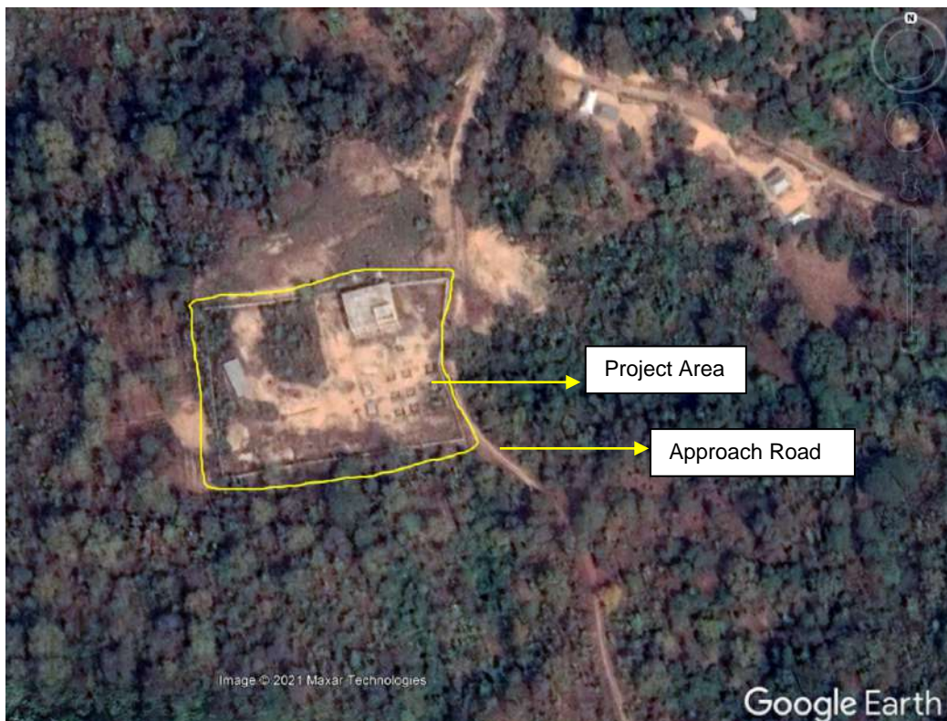
S/S Site in 2021 – Construction Work Under Progress
