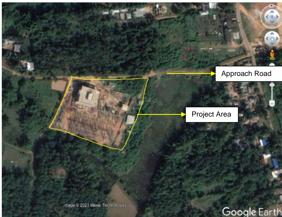
S/S Site in 2021 – Construction Completed
