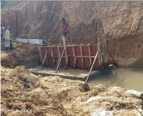
Retention Wall at 132 / 33kV Belonia SS
