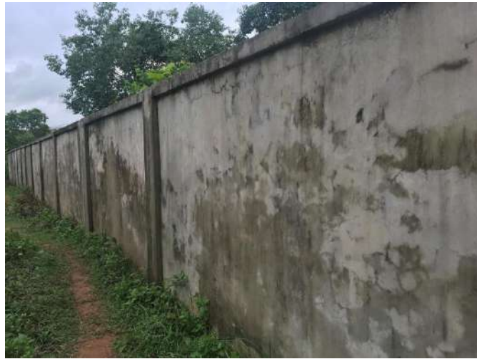
Boundary Wall - Nidaya S/S
