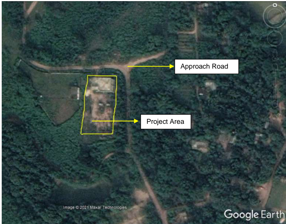
S/S Site in 2021 – Construction Work Completed
