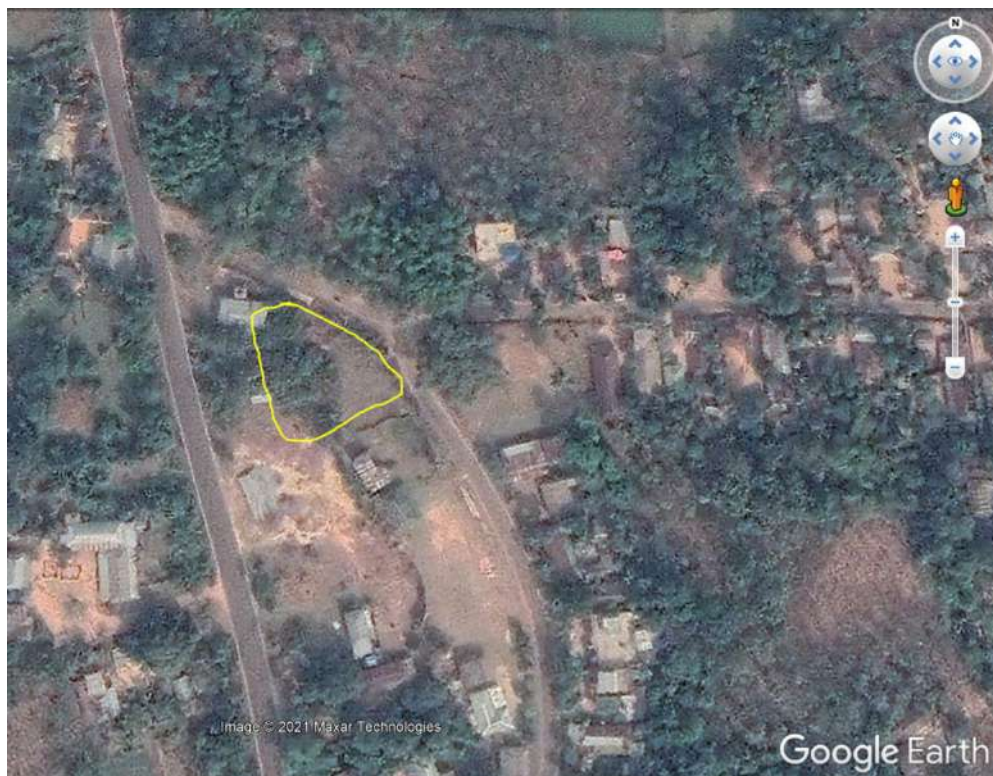
S/S Site in 2021 – Construction Work is Not Started.
