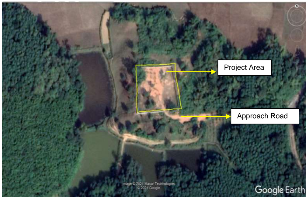
S/S Site in 2021 – Construction Work is Under Progress
