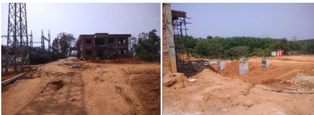
Gokul Nagar S/S Construction Site - Control Room Building
