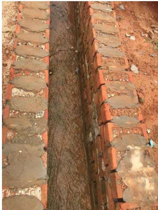
Drainage System Implementation – Gokul Nagar S/S
