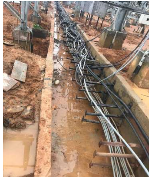
Transformer Erection (Left) and Cable Trench Construction (Right) in Rabindra Nagar S/S
