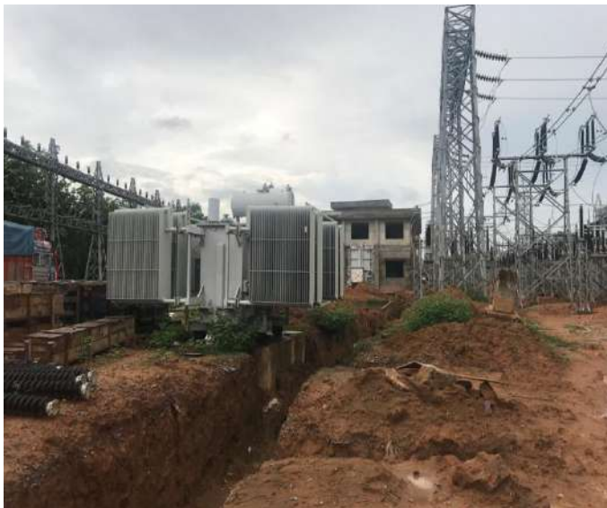
Transformer Erection (Left) and Cable Trench Construction (Right) in Rabindra Nagar S/S
