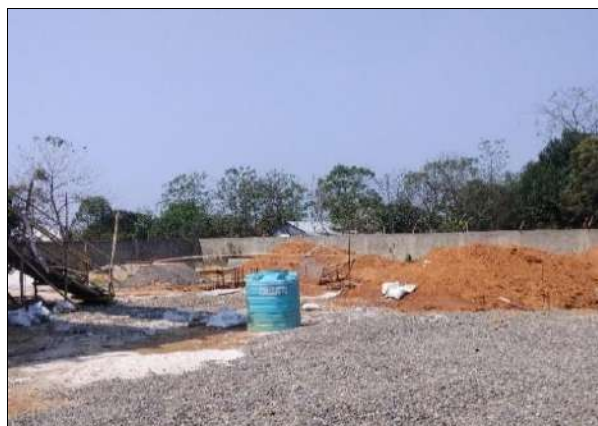
Mungiakami S/S construction site – Tower Foundation Work (Left) and CRB (Right)
