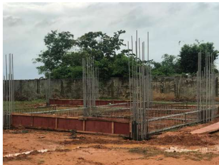
Nidaya Electric S/S - Construction Site
