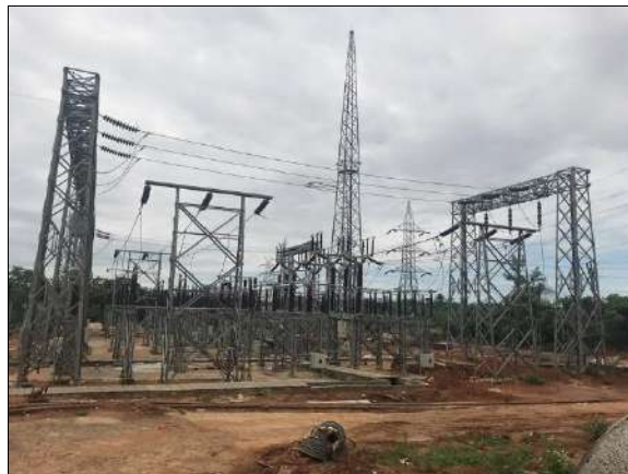
Gokul Nagar S/S construction site Tower Erection
