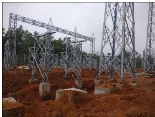
Barkathal S/S - Tower Erection
