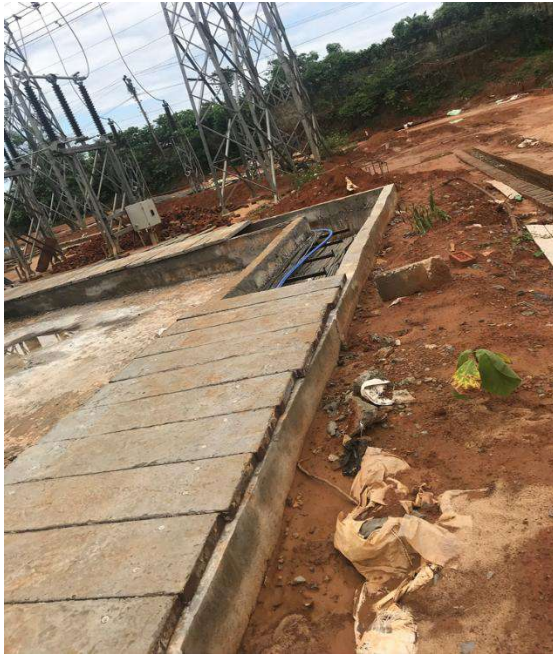
Cable Trench Construction Under Progress (Left) and Retaining Wall (Right) at Gokul Nagar S/S
