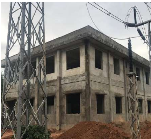
Substation Control Room Building Construction
