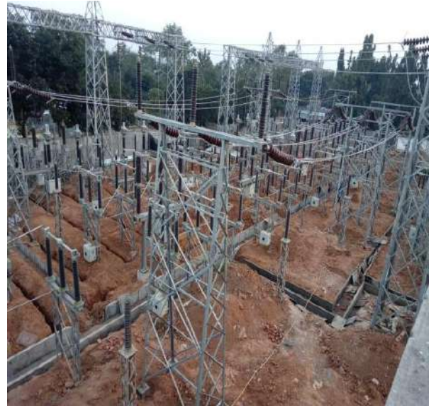
Foundation Work and Erection of Tower at Rabindra Nagar S/S
