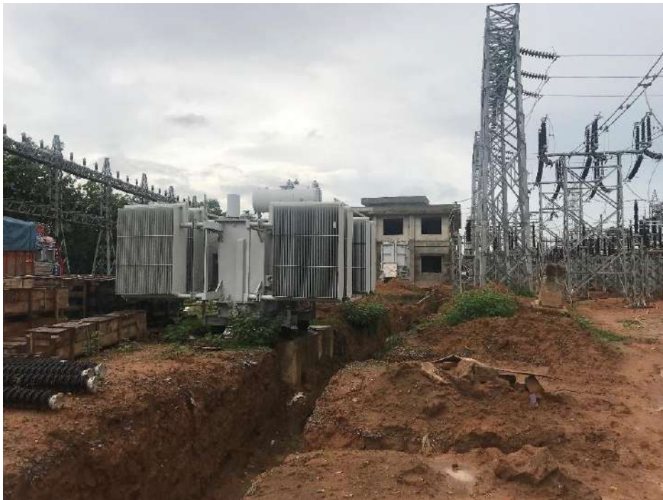
Transformer Erection with Oil pit in Progress – Rabindra Nagar S/S
