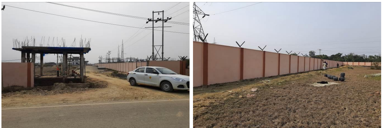
Boundary Wall and Gate at 132/33 kV Sarupathar Substation
