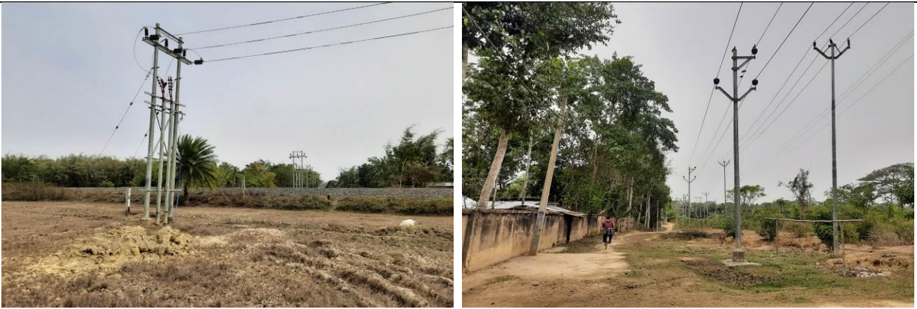
Route of the Line
