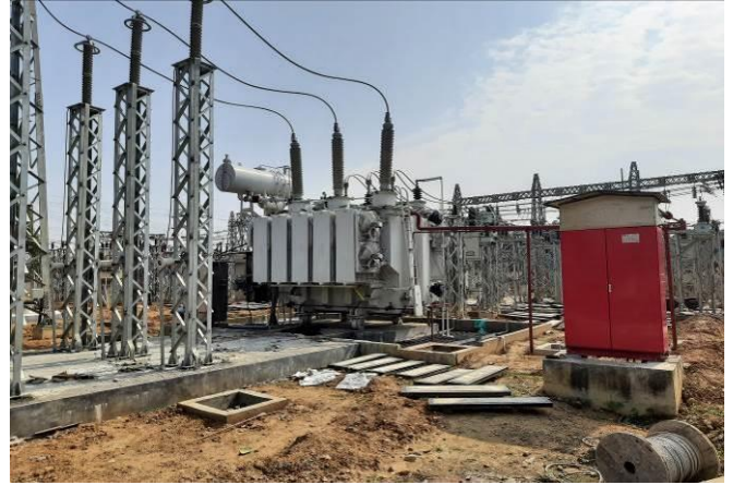
Oil Spill Containment Systems at 132/33 kV Sarupathar and Teok S/S
