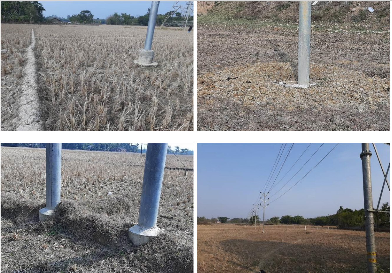
Levelled Sites after Erecting Poles
