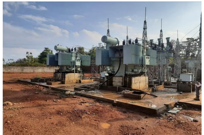
Oil Spill Containment Systems at 33/11 kV Hatimurah-II and Mailu S/S
