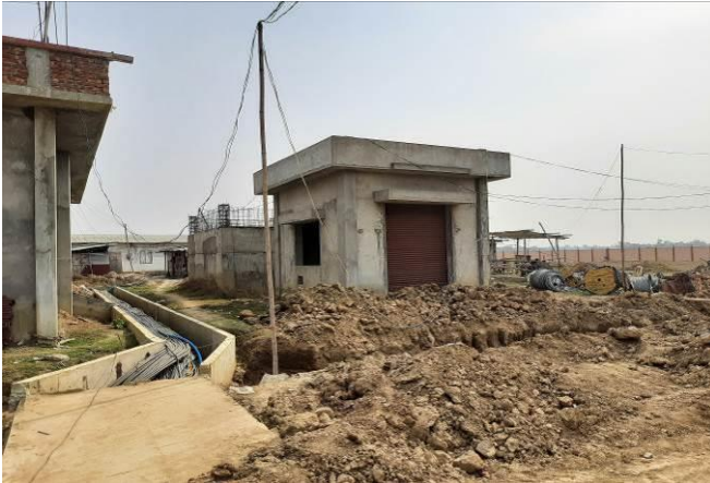
Fire Fighting Pump House, Water Tank, Cable Trench at 132/33 kV Sarupathar S/S
