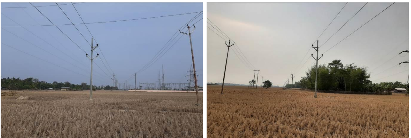
Route of the Line
