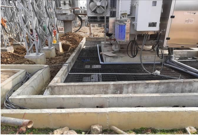
Oil Spill Containment Systems at 132/33 kV Sarupathar and Teok S/S
