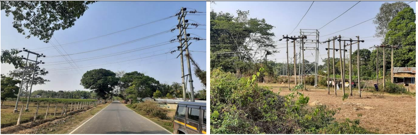
Route of the Line
