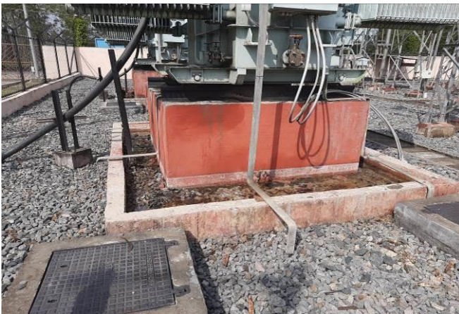
Oil Spill Containment Systems at 33/11 kV Hatimurah-II and Mailu S/S
