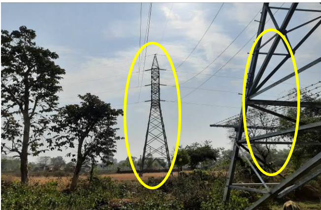
Tapping Tower and Tower No. 1/0
