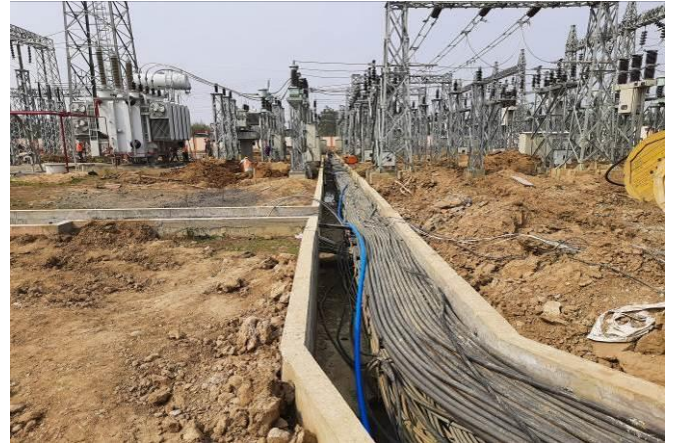
Fire Fighting Pump House, Water Tank, Cable Trench at 132/33 kV Sarupathar S/S
