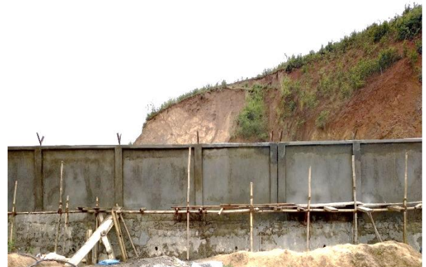
RRM Wall at 33/11kV Top-Khongnangkong
