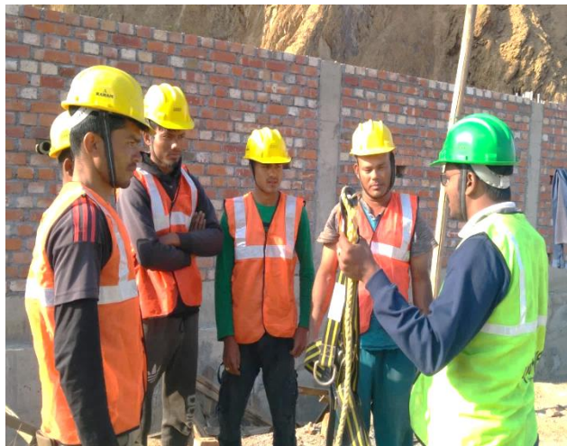
Safety Training at 33/11 kV Top Khongnangkong
