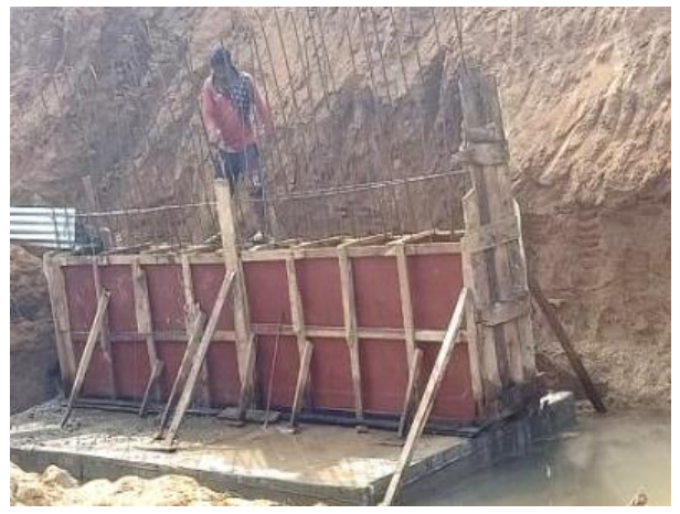
Retaining Wall at 132/33 kV Belonia
