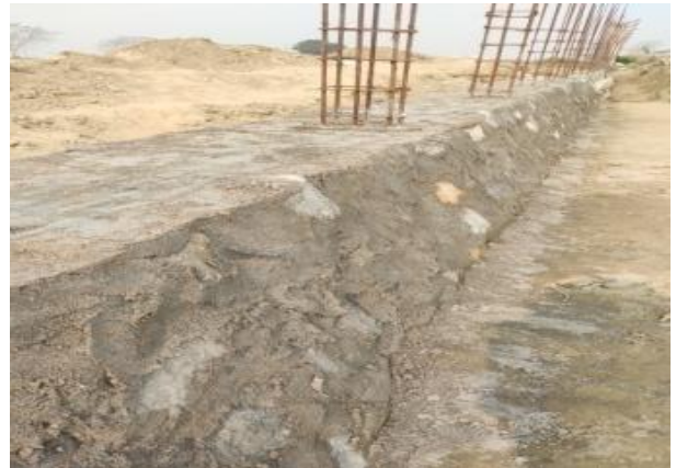
RRM Wall at 132/33 kV Hazo New,
