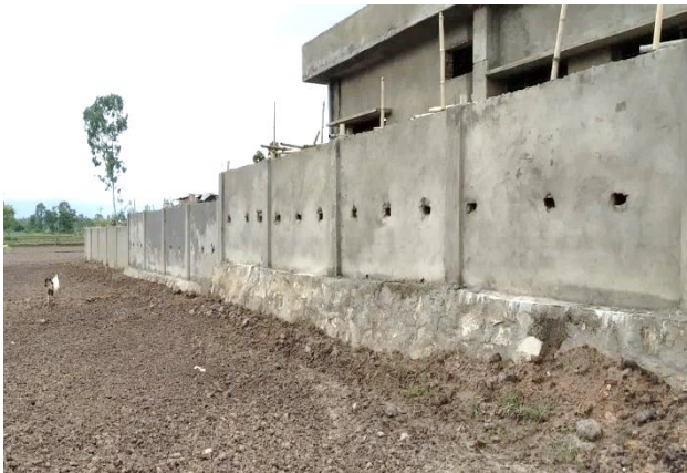
RRM Wall at 33/11kV Hiyangthang
