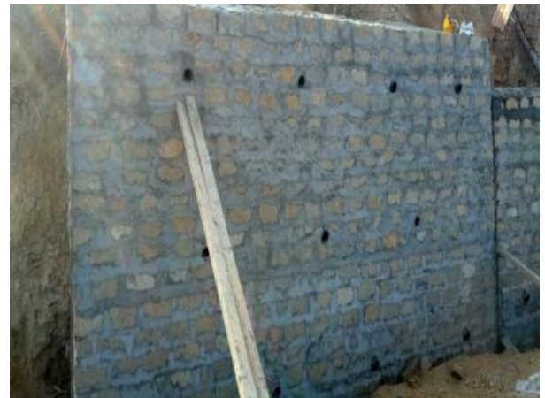
RRM Wall at 33/11 kV South Bungtlang
