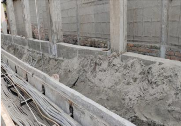
RRM Wall at 33/11 kV Domdoma Hazo,
