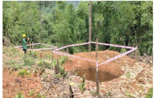
Barricading of Excavated Tower Pit Area of 132 kV West Phaileng-Marpara Line
