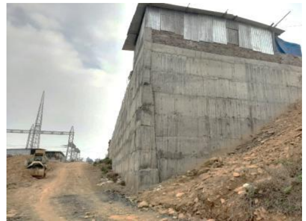
Completed Retaining Wall at 132/33kV New Secretariat complex Substation
