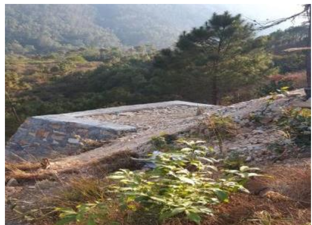
Retaining Wall at 200 kV New Shillong Section at AP 76
