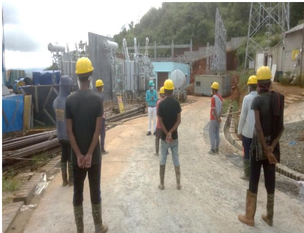
Safety Training at 220/132 KV New Shillong (GIS) substation
