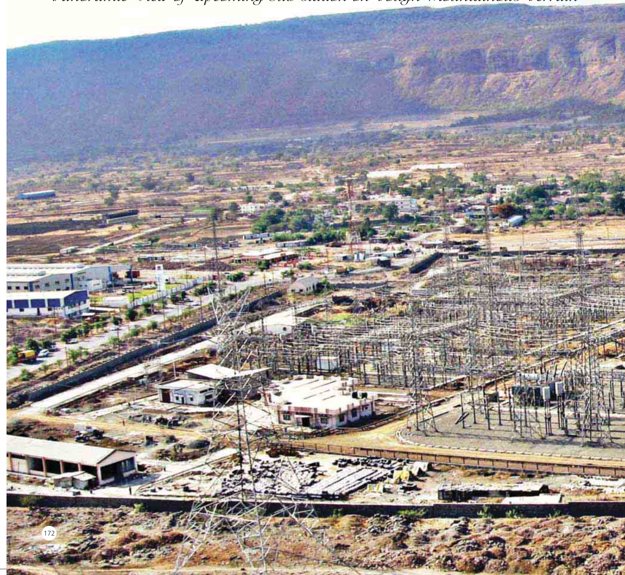
Panoramic View of Upcoming Sub-station on Tough Mountainous Terrain
