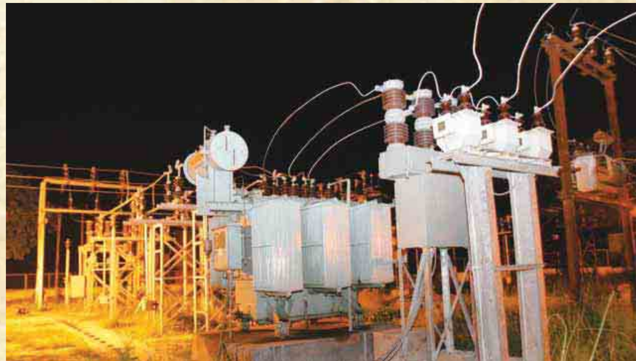
Work done under APDRP in Bihar
