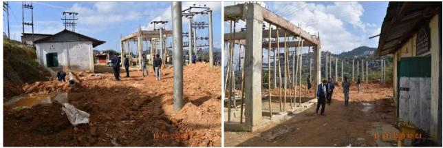
Refilling of excavated soil to avoid Soil erosion
