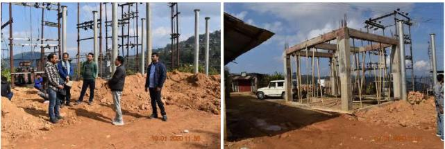
Refilling and leveling work at new 33/11 kV Substation at Longleng Town
