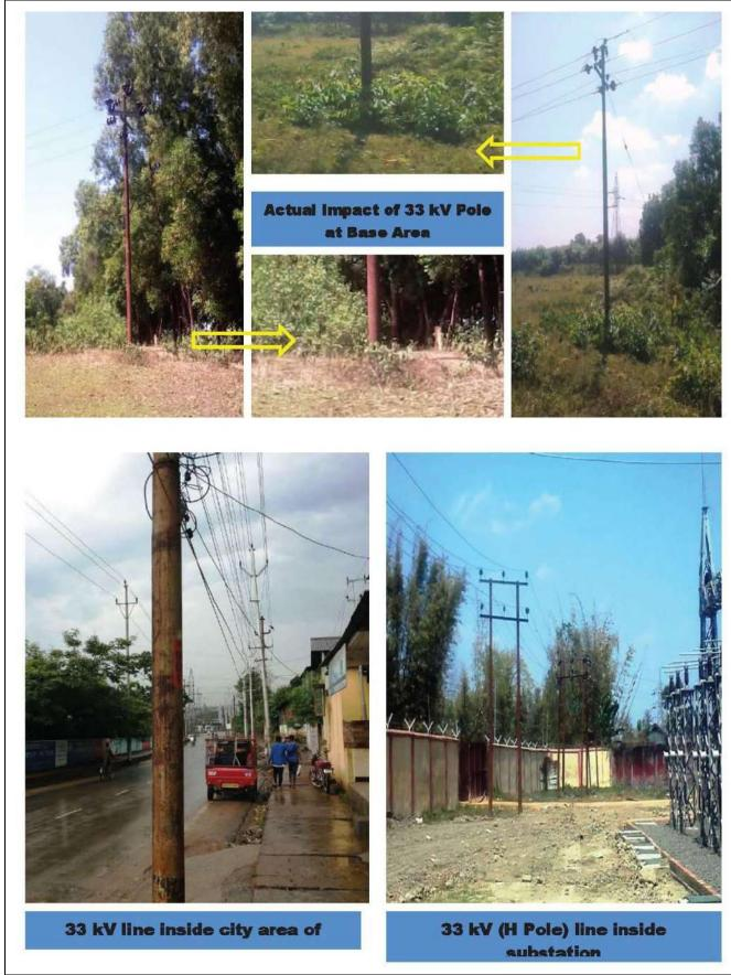
Figure 4.8: 33 kV Lines (Single & H Pole) Depicting Base Area Impact
