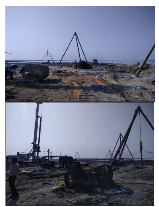
Pile foundation work at Brahmaputra river for construction of 132 kV Rupai-Chapakhowa Electric Line
