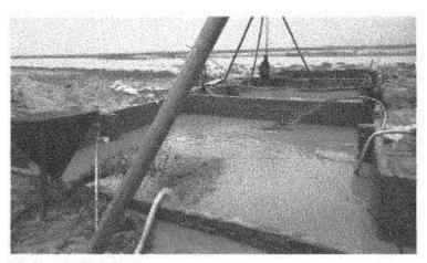
Fig. Bentonite Mixing Tank
