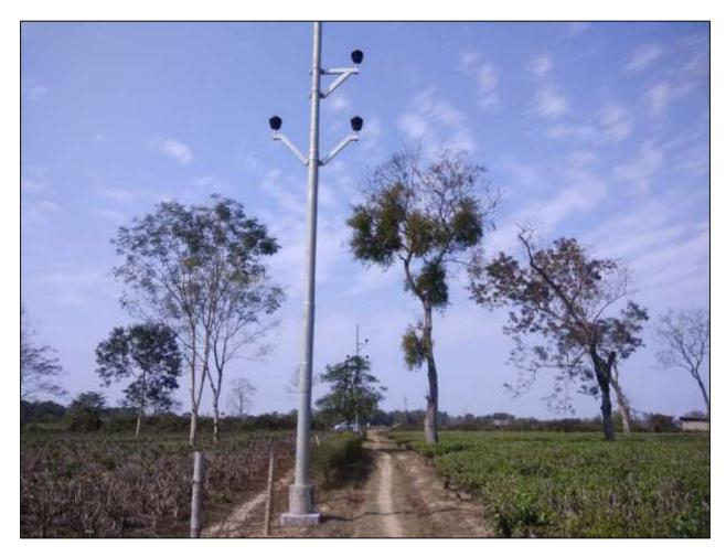
FIGURE 5-2 A PHOTOGRAPH SHOWING POLES OF BEHIATING-BOGIBIL 33 KV LINE IN WHICH A TREE IS
