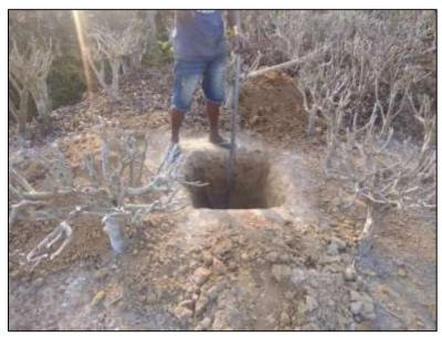
A photo showing excavation for construction of a pole for 33 kV Dibrugarh-Romai distribution line
