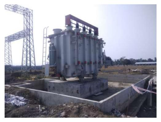
Provision for oil spillage prevention at Silapathar New substation
