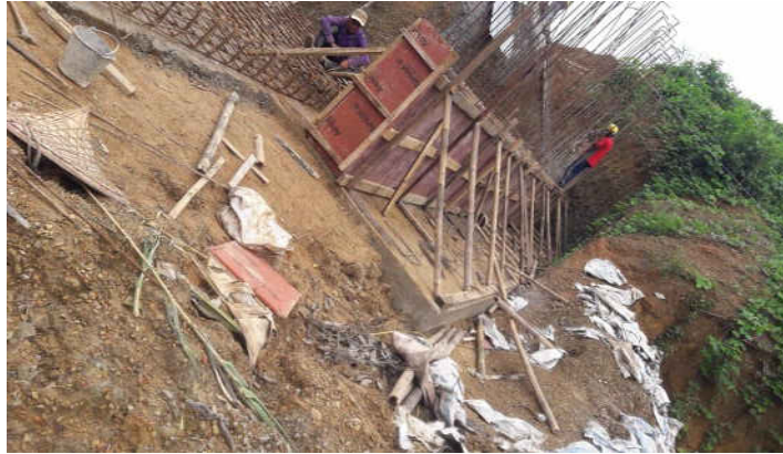
Figure 5-10 RCC Retaining wall construction at 132/33kV Marpara S/S
