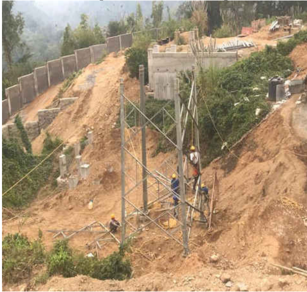
Figure 5-5 Erection work at 132/33 kV Marpara S/s and Casting at AP-22/0 W.Phaileng – Marpara T/L
