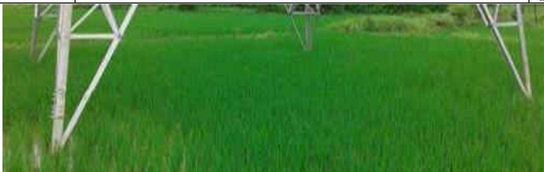
Figure 5-6 132 kV Tower Base (TL) Showing Impact on Agricultural Land and Crop
