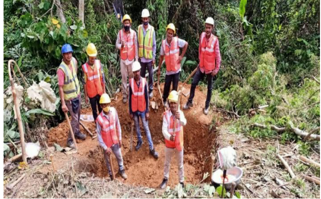
Safety induction training at 132kV W.Phaileng-Marpara TL
