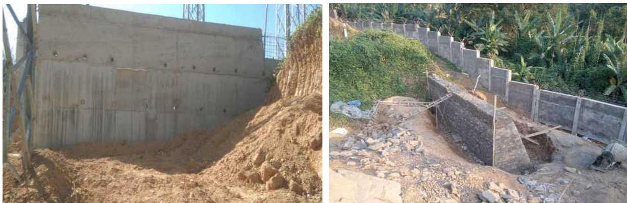
Figure 5-11 Erosion Control Measures
