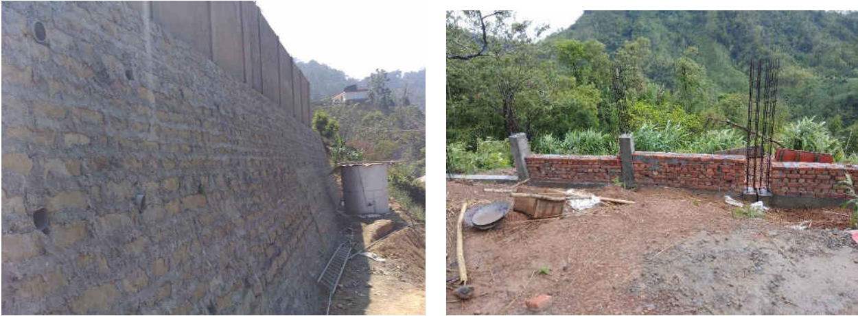
Figure 5-12 Erosion Control Construction
