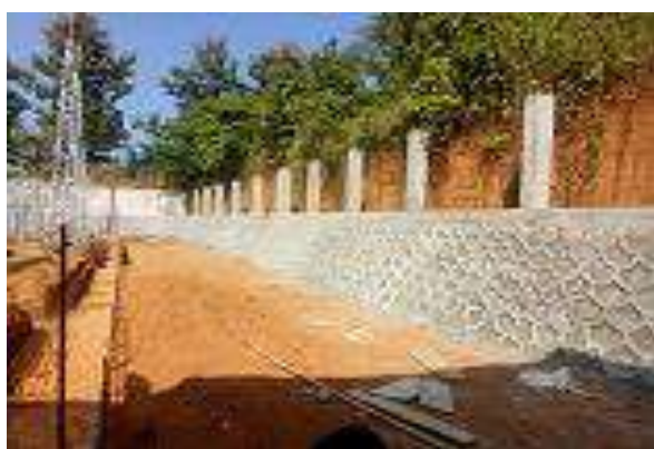
Figure 5.3 Retaining wall at 33/11 kV Raksambre
