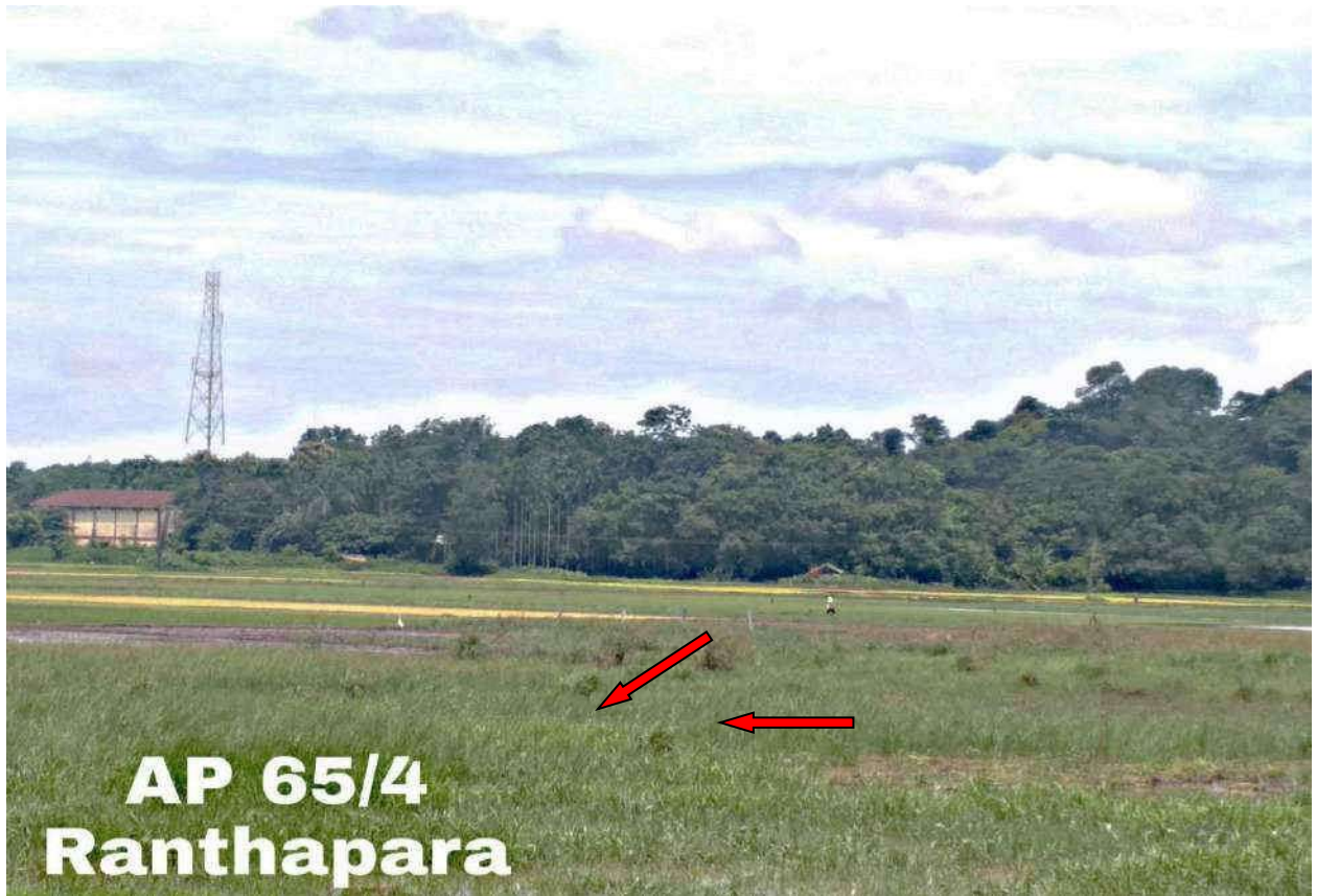
Tower footing (arrow)
