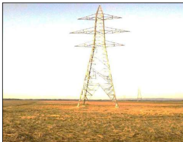
Figure 5.5 Construction during lean period
