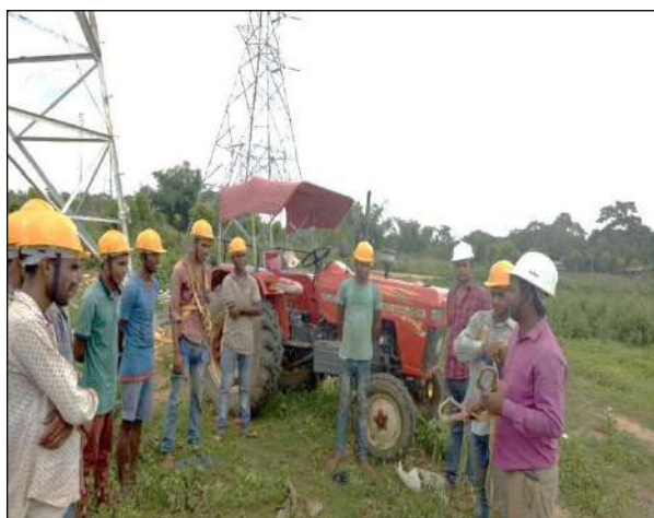
Figure 5.4 Use of Tractor for Stringing
