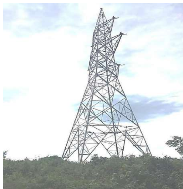
Figure 5.1 Tower installed at AP 72/0 with 9 m extension
