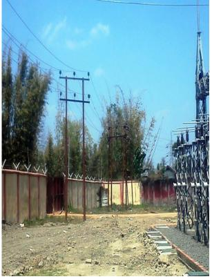
33 kV (H Pole) line inside substation
